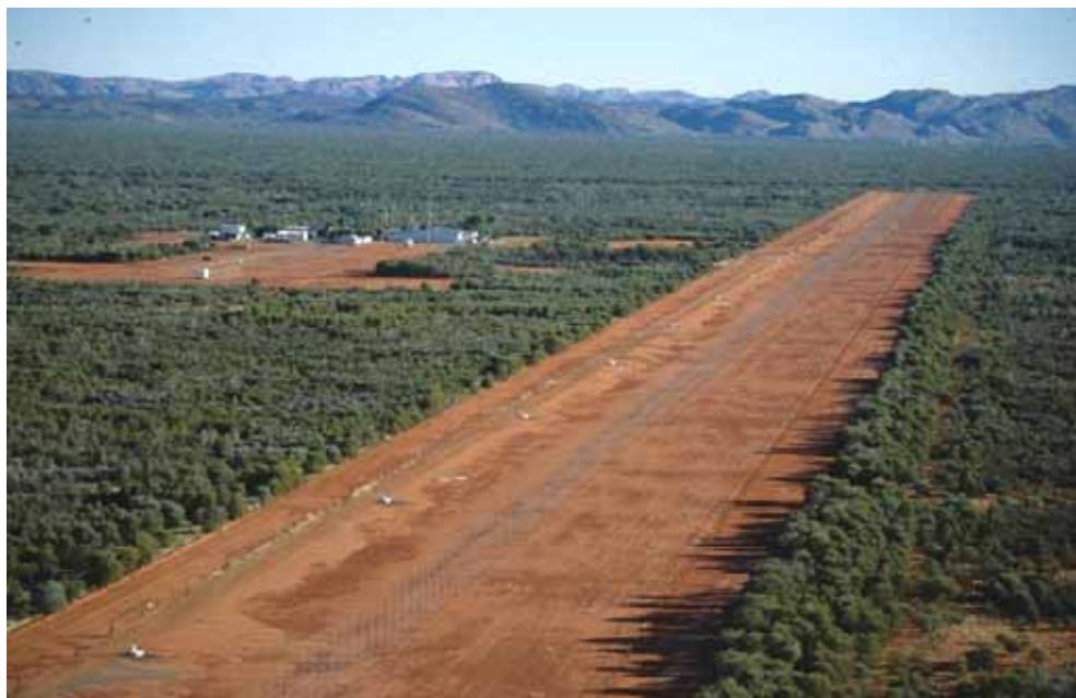
Fig. 2. Aerial view of the 2.8 km receiving array of the Australian Jindalee skywave radar, operational since 1982.
