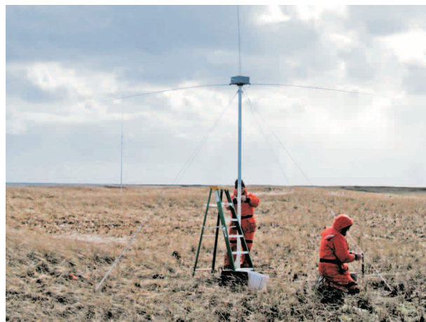
Figure 3. Picture of 5 MHz long-range SeaSonde. The receive antenna is shown in the foreground on the right. The transmit antenna is shown in the background on the left. Technicians installing the radar are shown for scale.
